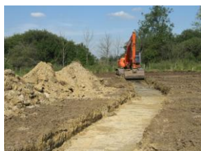
Backfilling the line of the drain with clay, Oxon.
