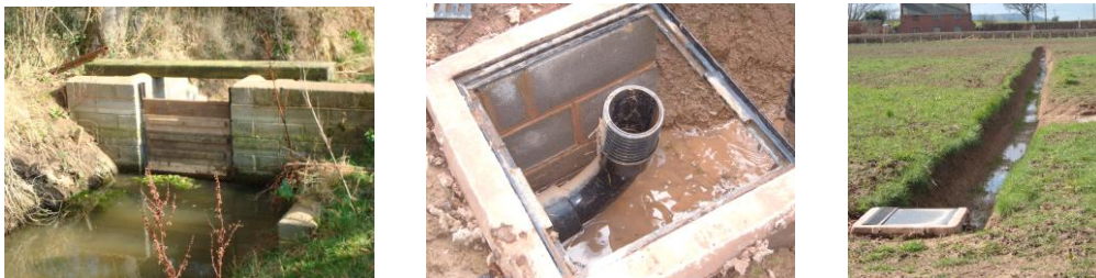
On this farm, a simple sluice has been placed mid way along a perimeter outfall ditch, and a right angled pipe control structure placed on one section of sub surface drainage pipe. A small length of the pipe was removed upstream of this to create a ditch/water retaining feature. This created some small scale wetness in a discrete area of the field. The remaining sub surface drainage system network downfield of this point was left in situ.
