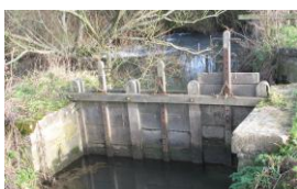
Historic water meadow sluice
