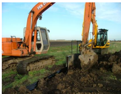
Installing a plastic membrane, Cambs
