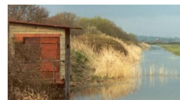
Modern pump house, Oxon.
