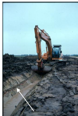
An excavator removing a section of sub surface tile drain, Oxon.
