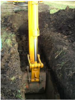
Inspection trench, Cambs.
