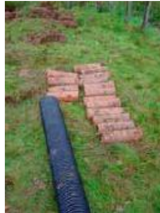
2. Clay tiles removed, and plastic pipe ready for installation
