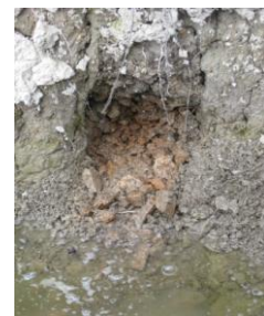
Gravel backfill exposed by excavations, Shrops.
