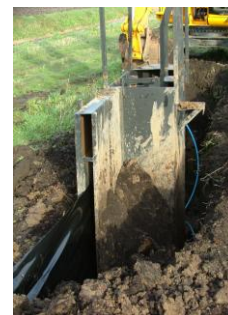
Plastic sheet dispensing from trenching rig, Cambs.
